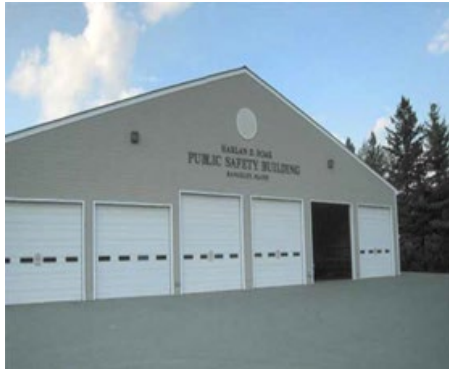
Rangeley's Public Safety Building
